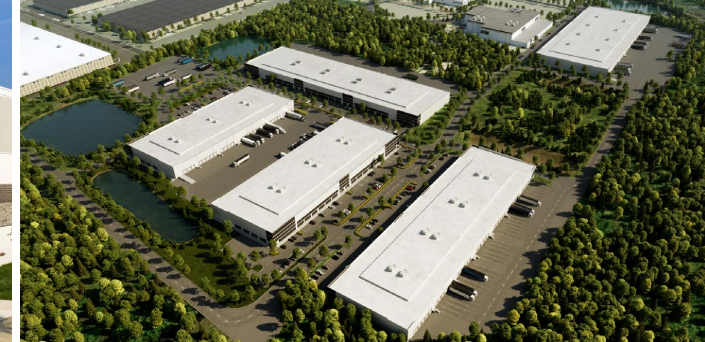
Northlake II 5-Building, 655,000 SF Industrial Park
