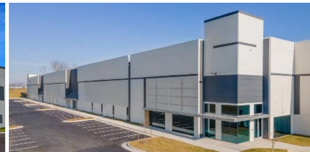
Parkway 66 High Bay Warehouse, Manassas, VA
